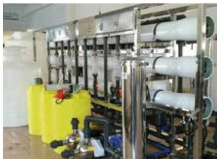
at a local semi-conductor company to recycle the rejected water from its Reverse Osmosis (RO) facility. 60 to 70 per cent of the RO rejected water will be recycled to replace part of the NEWater supply
